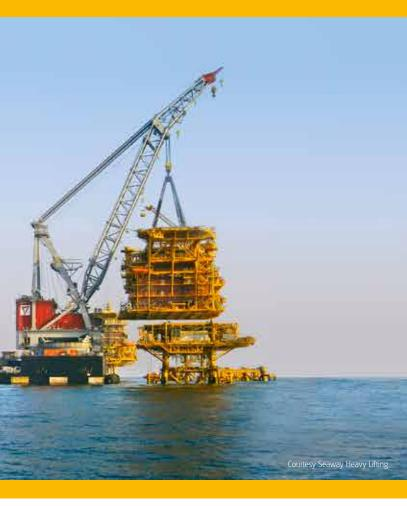
and the base frame also had ballast compartments. We had to ballast the barge and the frame, operate the crane and tugger winches and the vessel ballasting system." And this proved quite demanding on the system, which actually crashed several times. "We basically overloaded the processors! But we all went away, regrouped and went back with lessons learnt from the first time. However, we are stretching the limits, there is no doubt."
